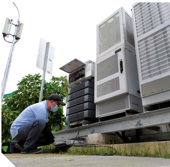
Engineer maintaining a mobile base station.
